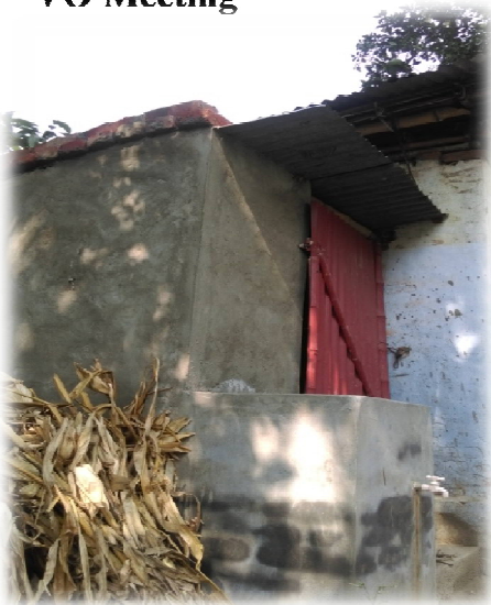
Toilet Construction in Sour Bazar
